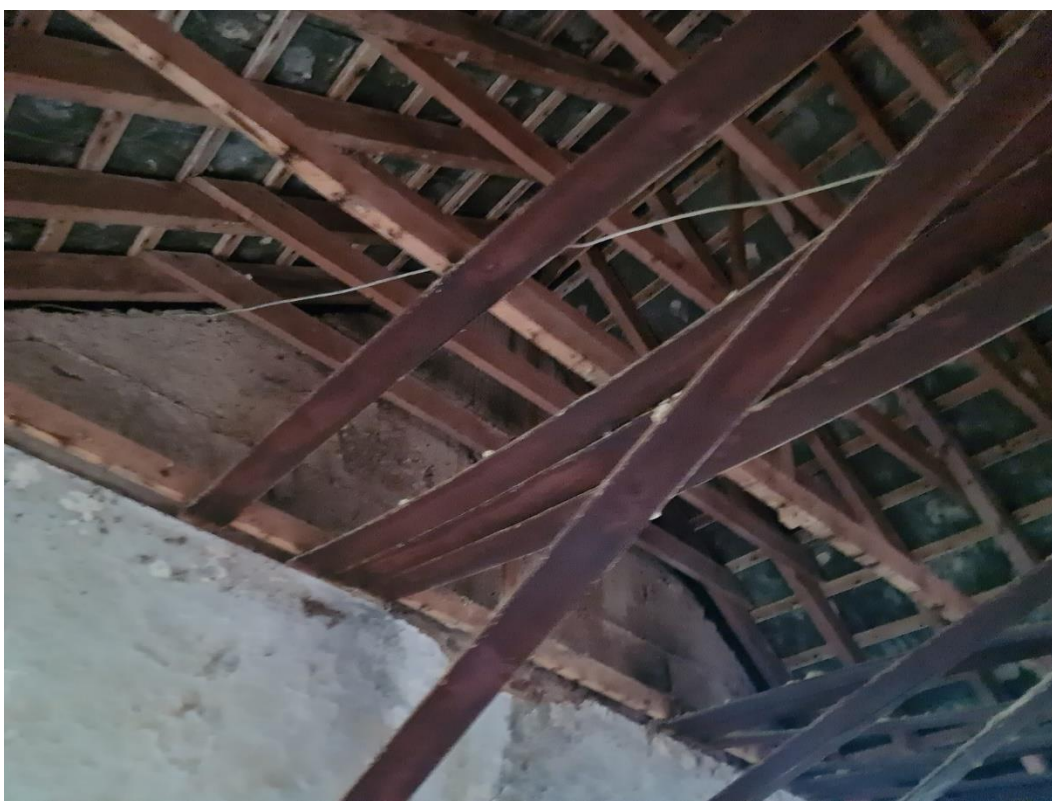
Plate 3: Structure 2. Internal view of dwelling. Quite a lot of light exposure
