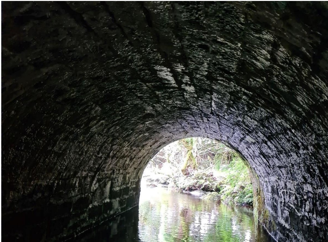
Plate 12: Structure 7. Joints are mortared.
