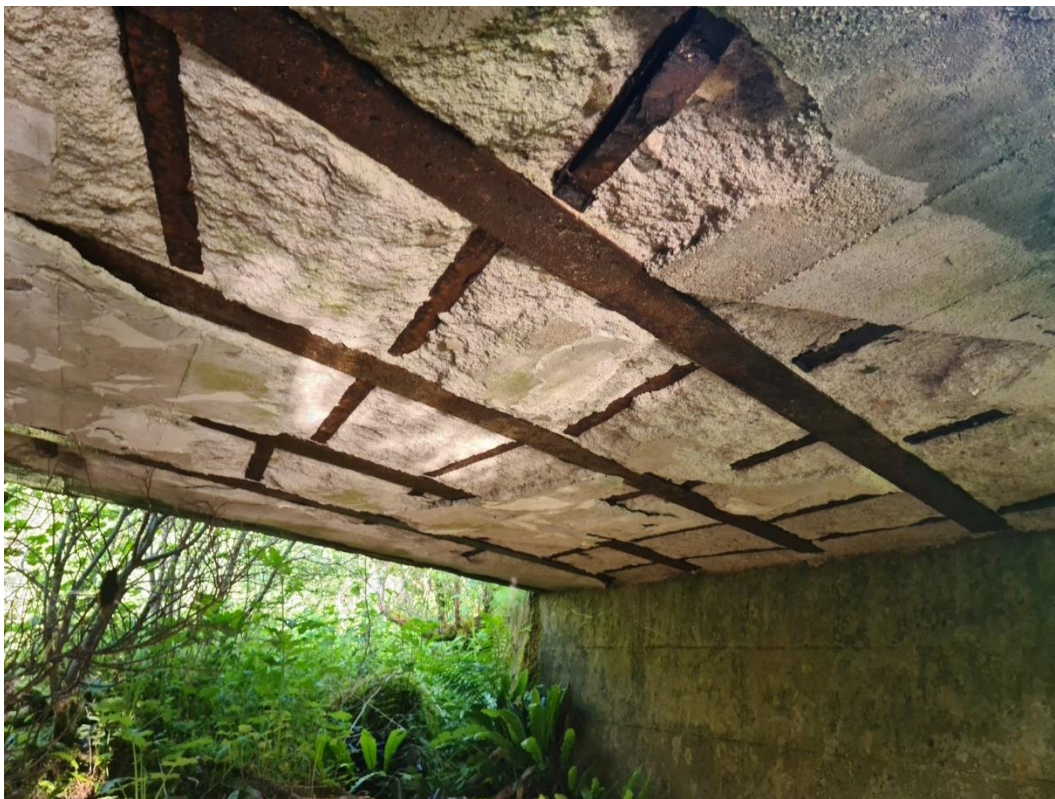
Plate 7: Structure 4. Concrete bridge
