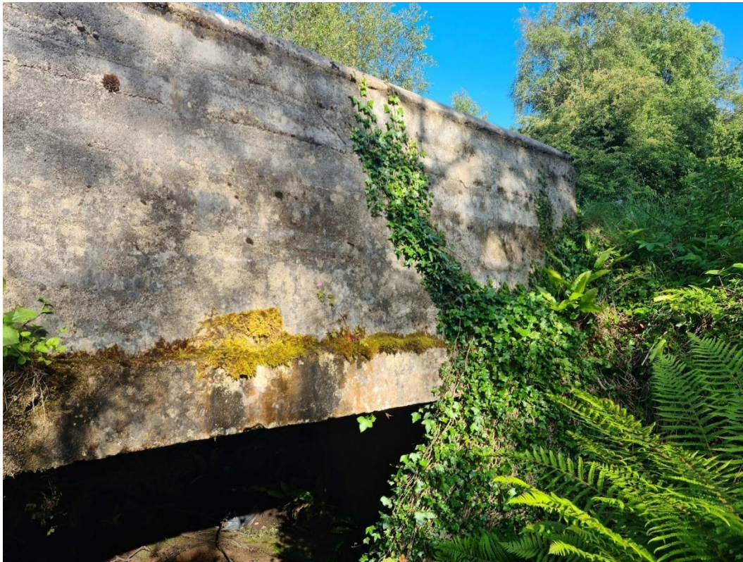
Plate 6: Structure 4. Concrete bridge
