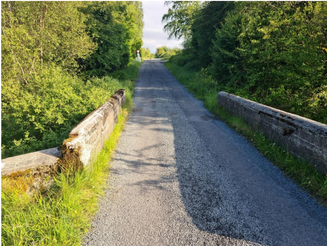
Plate 5: Structure 4. Concrete bridge
