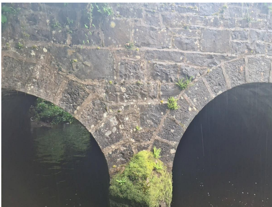
Plate 11: Structure 7. Bridge to SW of proposed site
