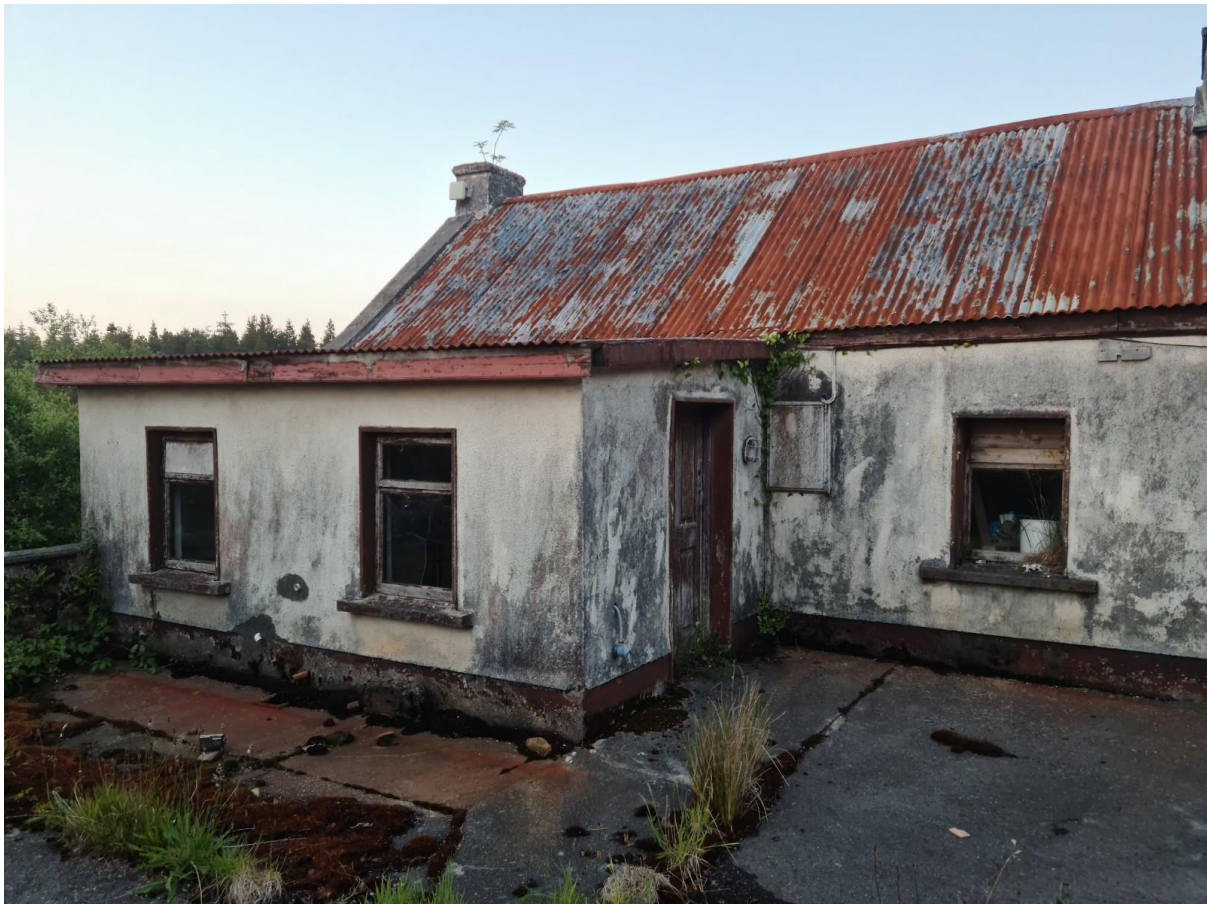
Plate 1: Structure 1. Derelict dwelling
